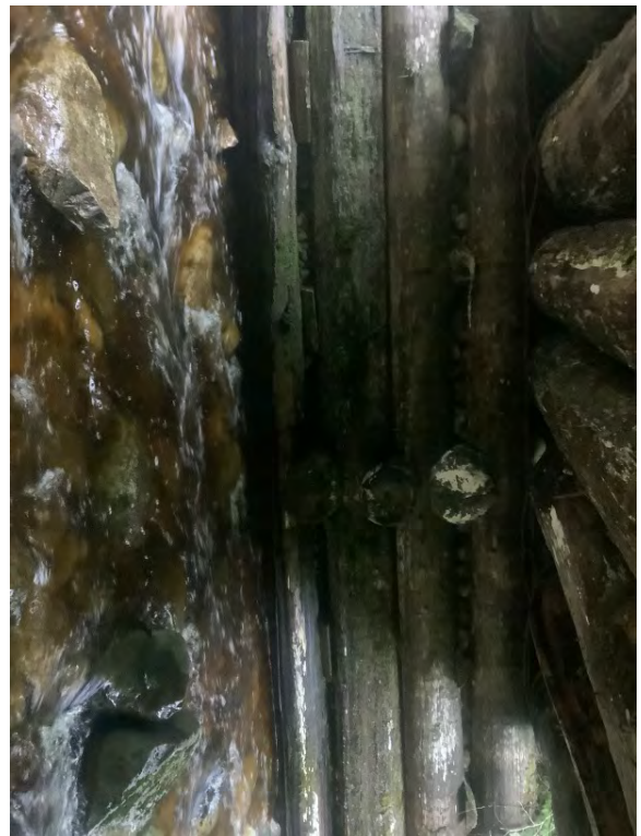
Left Bank Abutment when facing downstream
