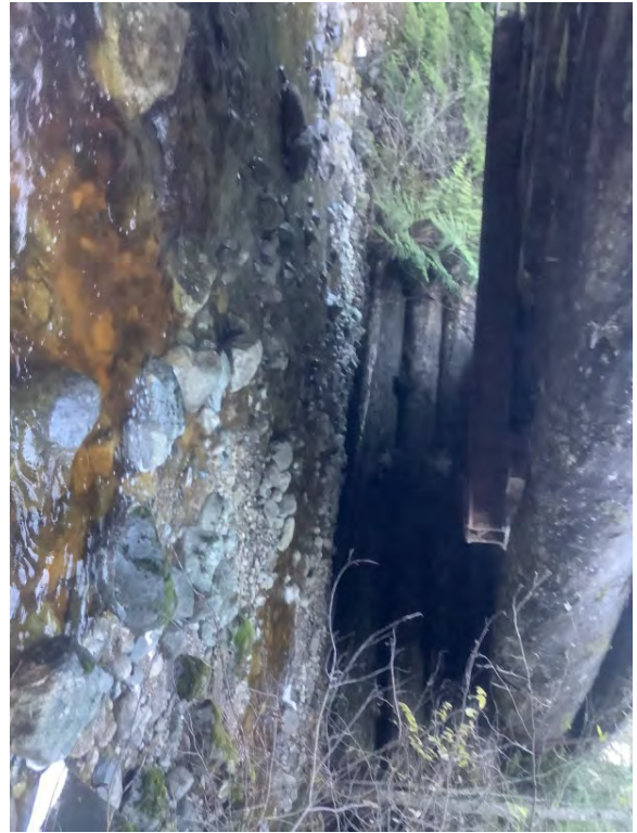
Right Bank Abutment when facing downstream
